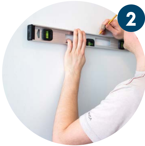
With a level plot the holes on a wall.
