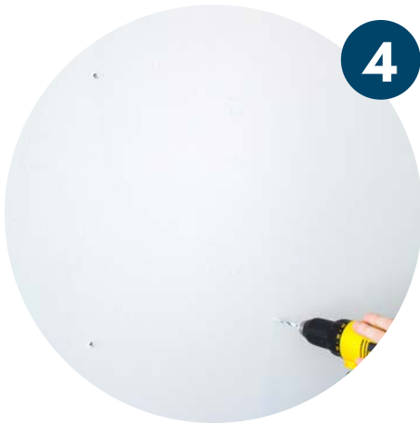
Drill pilot holes for the drywall plugs
