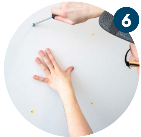
Screw in bottom thread onto the wall
