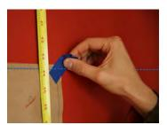
On the right side, slide the template up or down to match. Once it's level, firmly tape the corner of the template to the wall.
