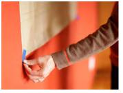
Exact spacing between the pegs is important, so make sure the template is stretched tight against the wall. Add tape to the bottom corners.
