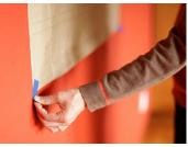
Exact spacing between the pegs is important, so make sure the template is stretched tight against the wall. Add tape to the bottom corners.
