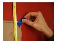
On the right side, slide the template up or down to match. Once it's level, firmly tape the corner of the template to the wall.
