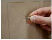
Use a peg to make a small hole at the center of each cross-hairs.
