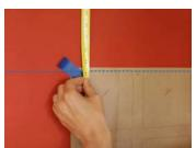
On the left side, measure the distance to the ceiling using the tape measure.
