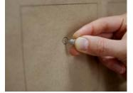
Use a peg to make a small hole at the center of each cross-hairs.
